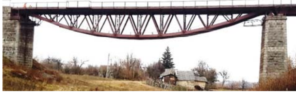
Fig. 1. General view of truss
