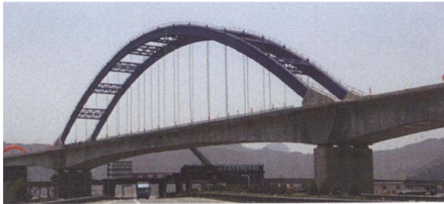
(a) Kuyang Bridge
