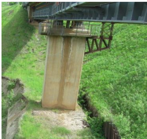
Figure 25. Leaching of cement paste
