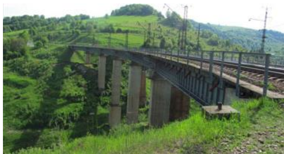
Figure 2. Steel-concrete composite viaduct in the mountainous terrain of the Carpathians
