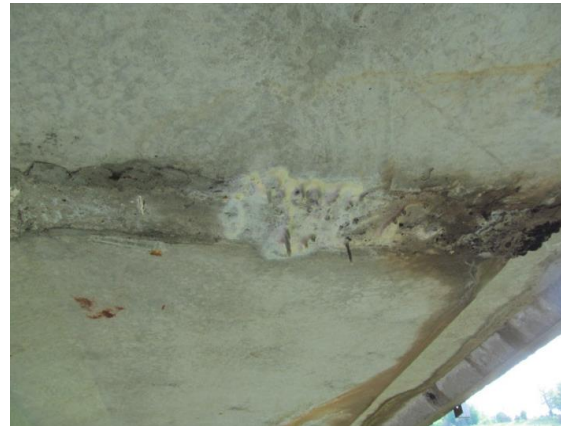
Figure 16. Leaching of cement paste
