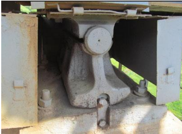
Figure 19. Undercutting of anti-creep teeth
