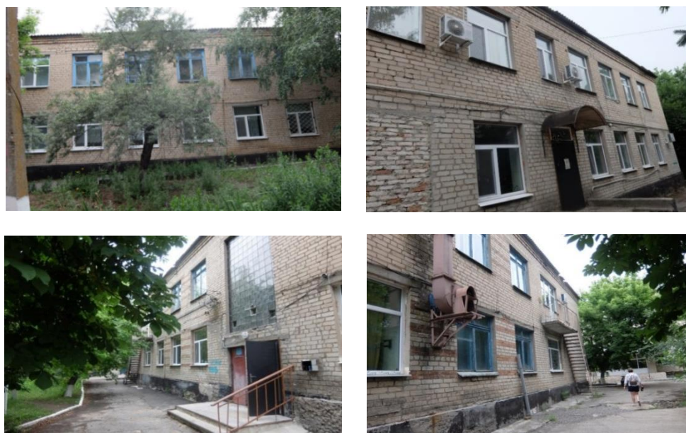
Figure 1. Appearance of the building facade
