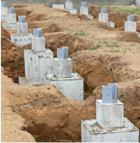
Figure 1. Monolithic column foundation
