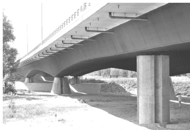
Fig. 7. The highway bridge over the Ostravice River in Ostrava, Czech Republic
