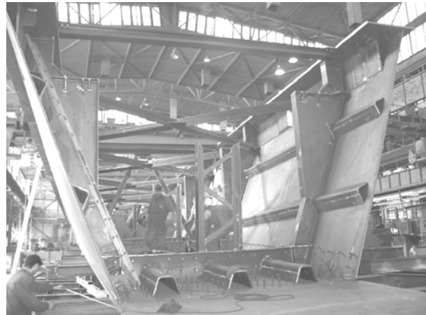
Fig. 9. The steel girders during assembly stage [4, 5]
