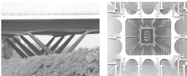
Fig. 5. The V-shaped bridge supports – general view and interior view of the supports [4, 5]
